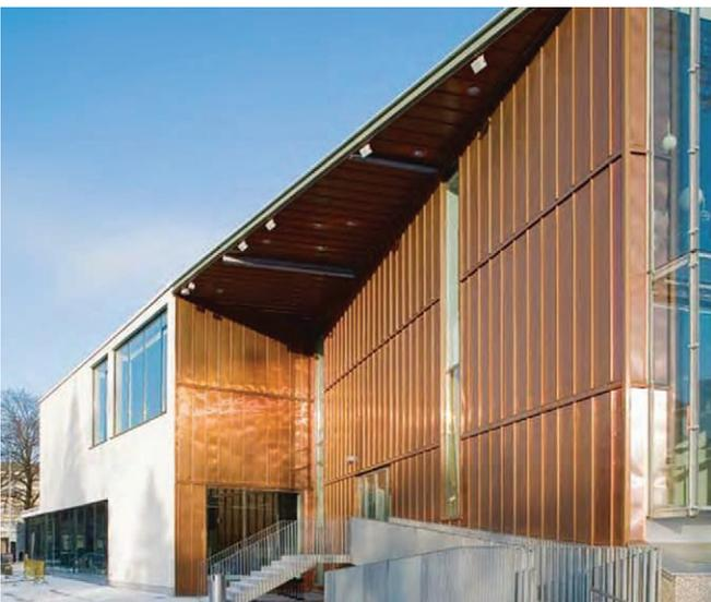
Aurubis' products for architectural applications such as facades and roofs use phosphorus deoxidised copper, designated Cu-DHP and complying with EN 1172:1997 – 'Copper and Copper Alloys: Sheet and Strip for Building Purposes'. This pure and natural material exhibits a unique range of characteristics and performance benefits including:
